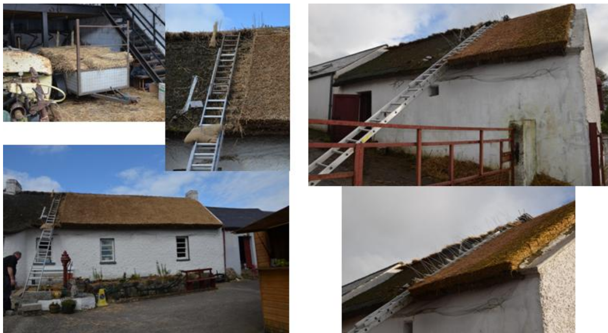
Thatching at Dan Winter's cottage
