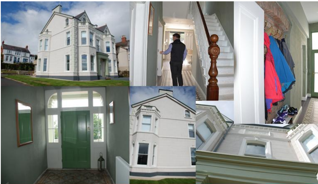
Princetown Road- after conservation works
