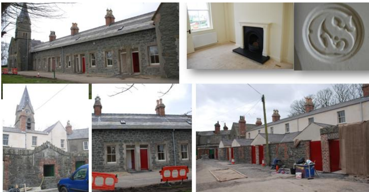
Conservation works at Shiel's Housing Killough
