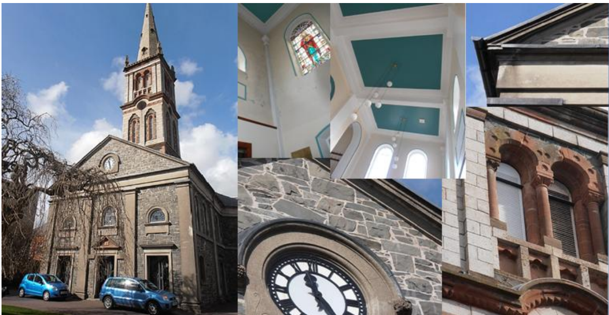
1 st Presbyterian Church Bangor – stone repairs
