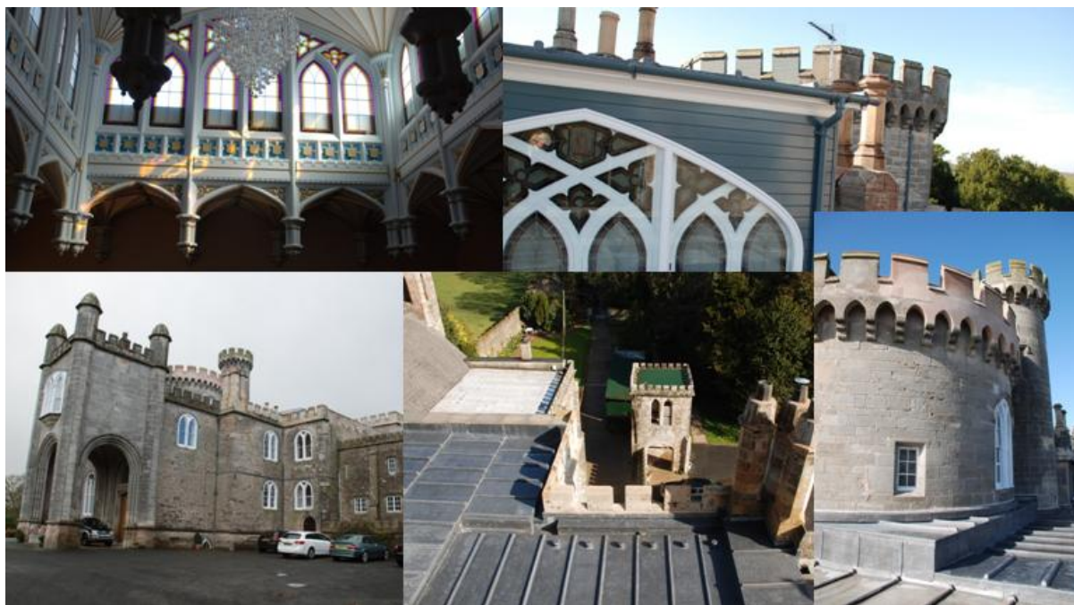
Killymoon Castle- roof repair works
